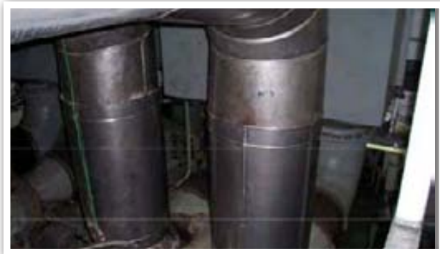
MMPP "Castilla" piping modification
